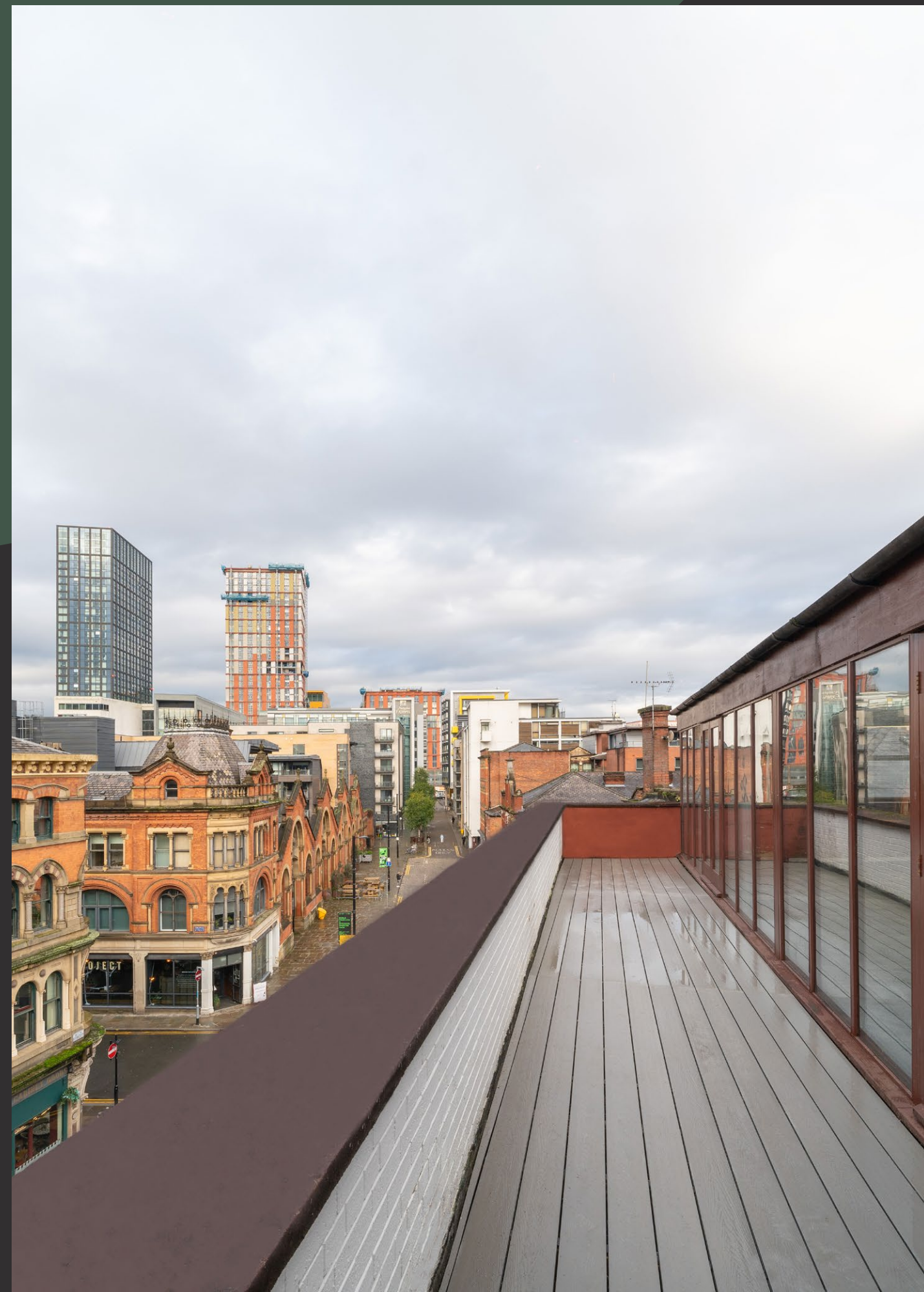
4TH FLOOR TERRACE
